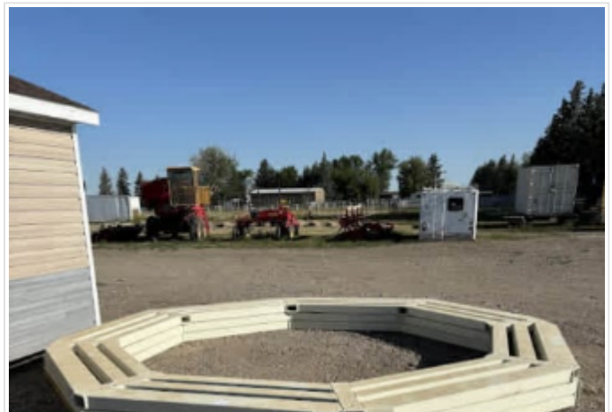
#5133A Bin Foundation
