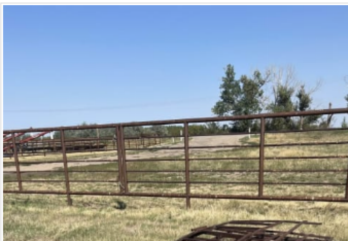
#4764B Feeder Panels
